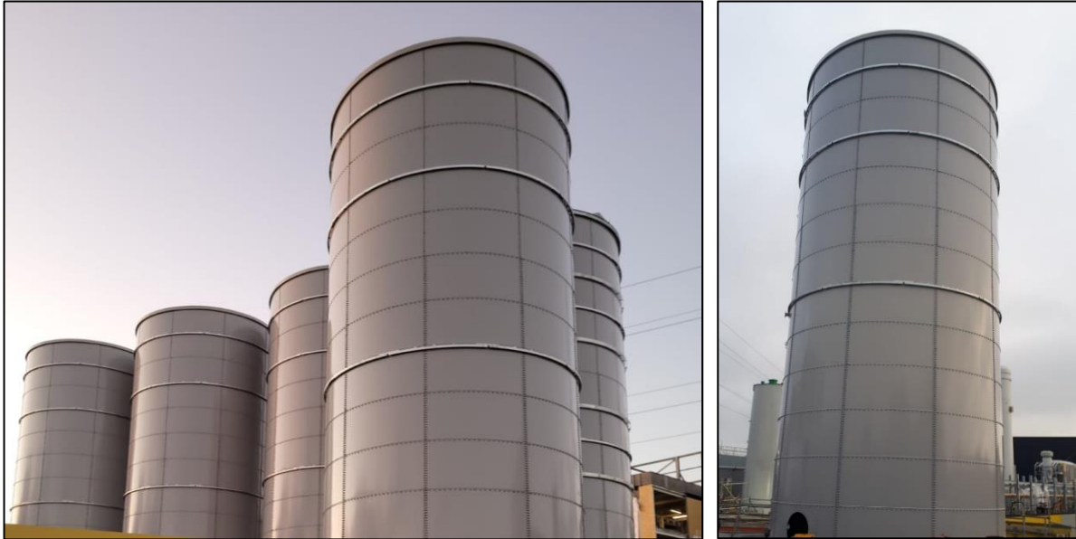
Left: 5no. Tanks Erected on Site Right: Tank No.1 nearing completion.
